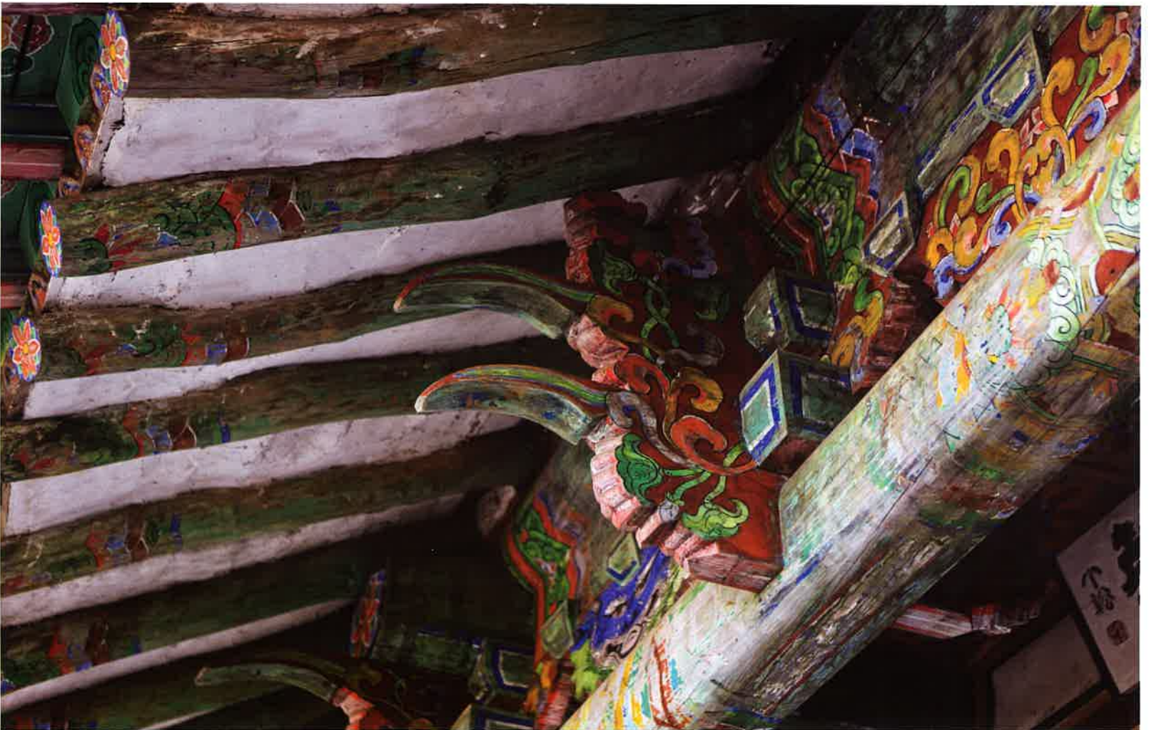
동금강암 앞면 주간포와 화반 / 東金剛庵 前面 柱間包·花盤 brackets between front columns and Hwaban, Tonggūmgangam
