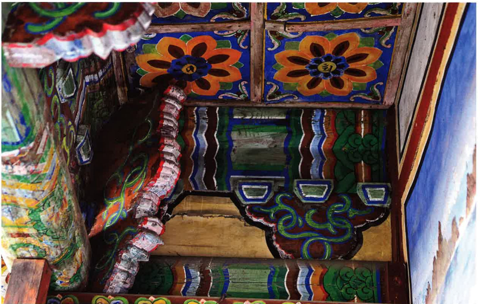
동금강암 뒷간 서쪽 측면 귀포 / 東金剛庵 退間 西側 耳包 western corner brackets of space with extra poles outside the inner fence, Tonggūmgangam
