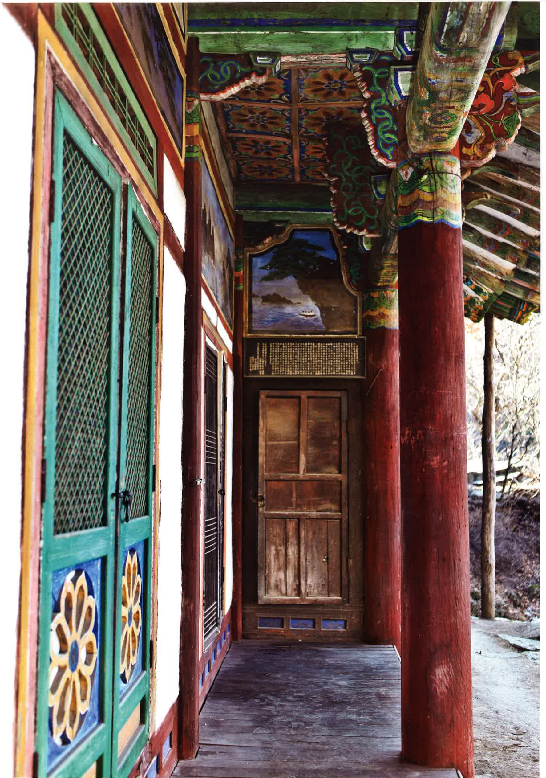
동금강암 뒷간 / 東金剛庵 退間 / space with extra poles outside the inner fence, Tonggungangam
