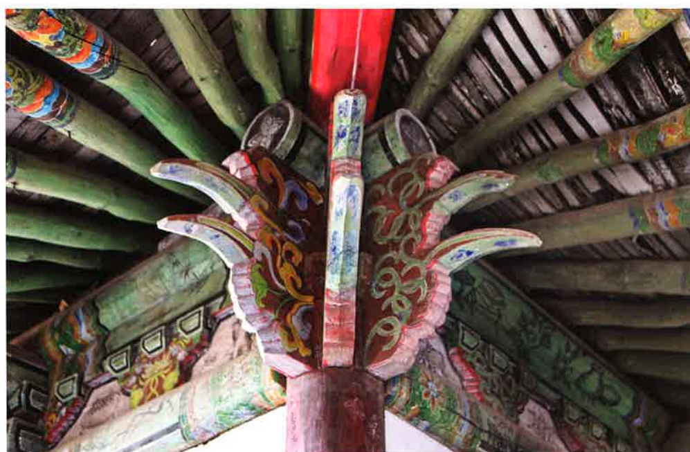
동금강암 뒷면 귀포 / 東金剛庵 後面 耳包 backward corner brackets, Tonggümgangam
