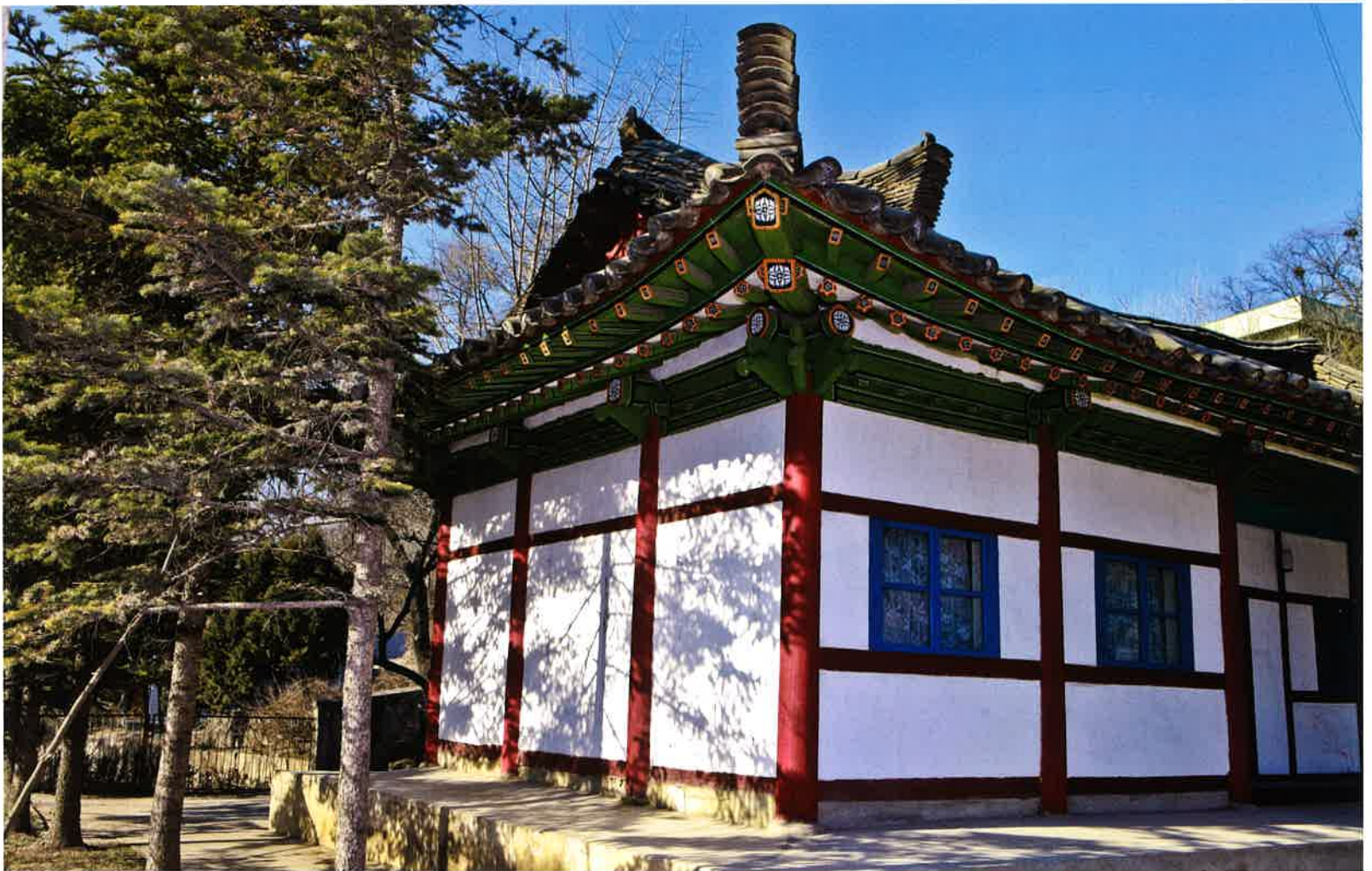
요사채 측면 / 寮舍齋 側面 / side, priest's residence
