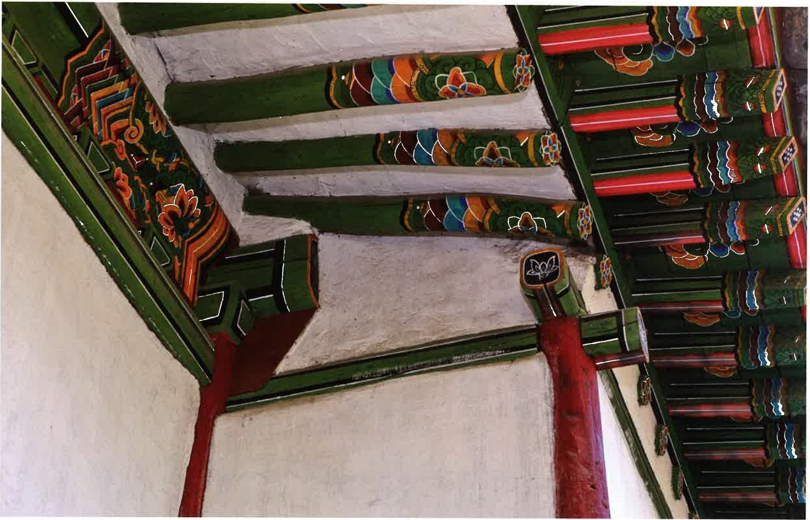
대웅전 뒷면 처마와 공포 / 大雄殿 後面 軒·拱包 / backward caves and brackets, Taeungjŏn hall backward caves and brackets, Taeungjŏn hall
