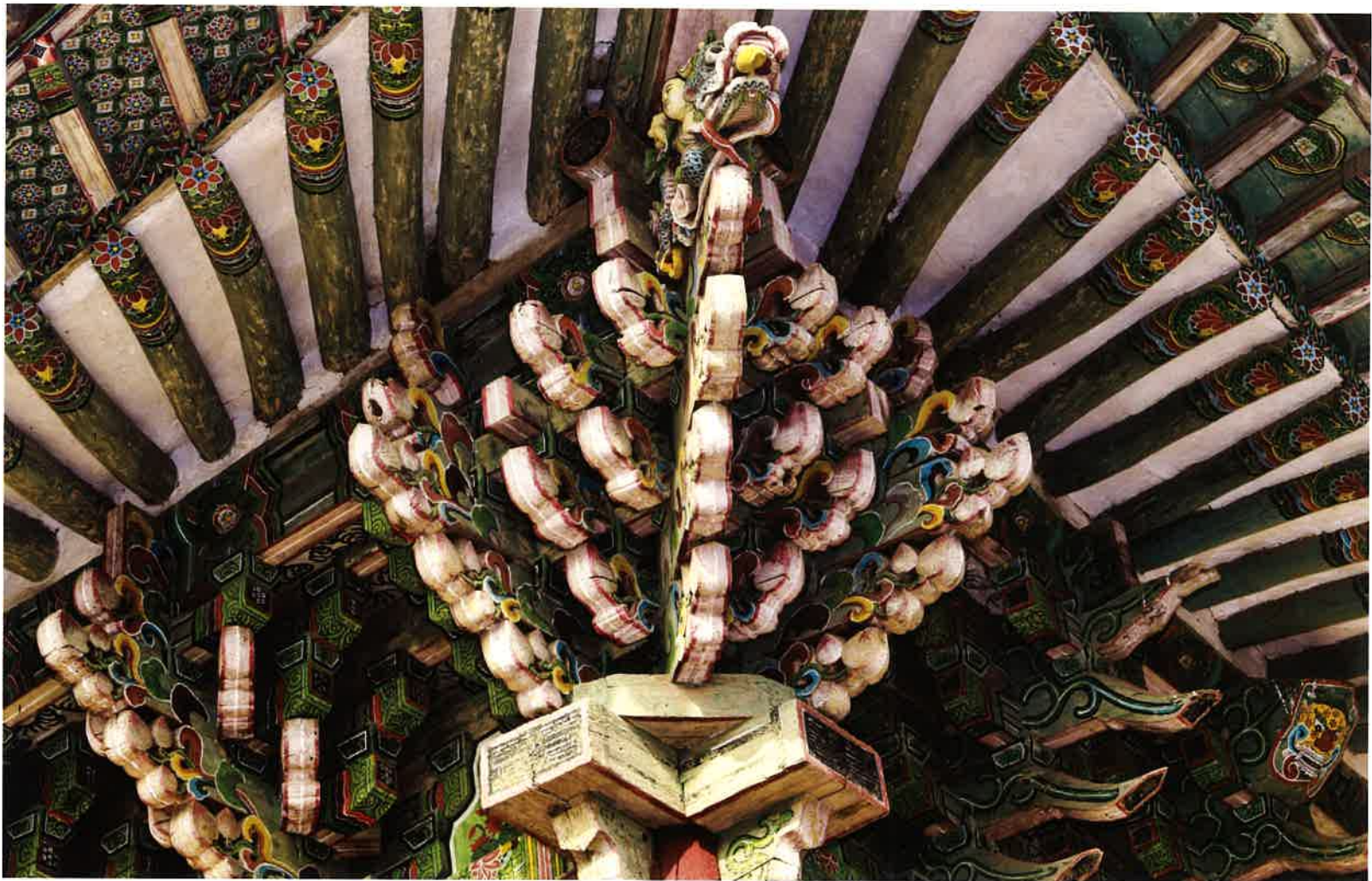
대웅보전 동쪽 추녀 / 大雄寶殿 東側 春舌 / eastern protruding corners of eaves, Taeungbojön hall
