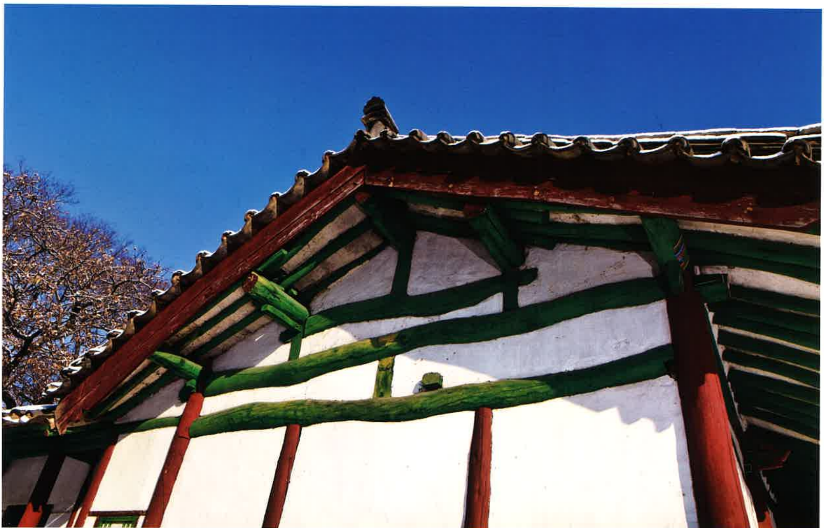
요사채 동쪽 측면 벽체 / 寮舍寨 東側 壁體 / eastern wall, priest's residence
