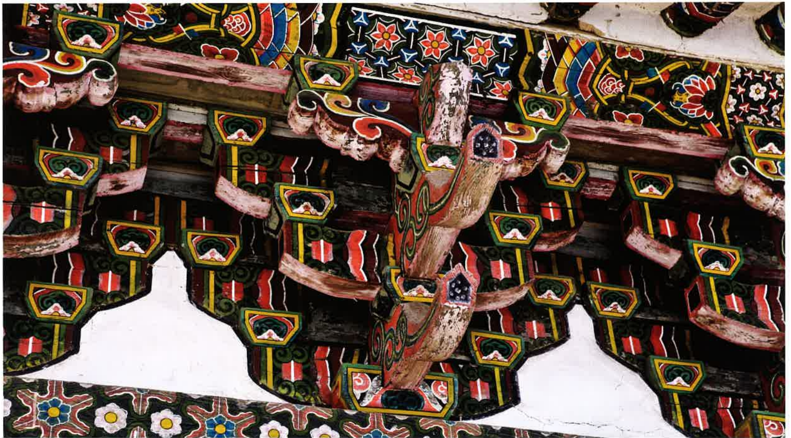
장경각 앞면 주간포 / 藏經閣 前面 柱間包 / brackets between front columns, Changgyōnggak hall
