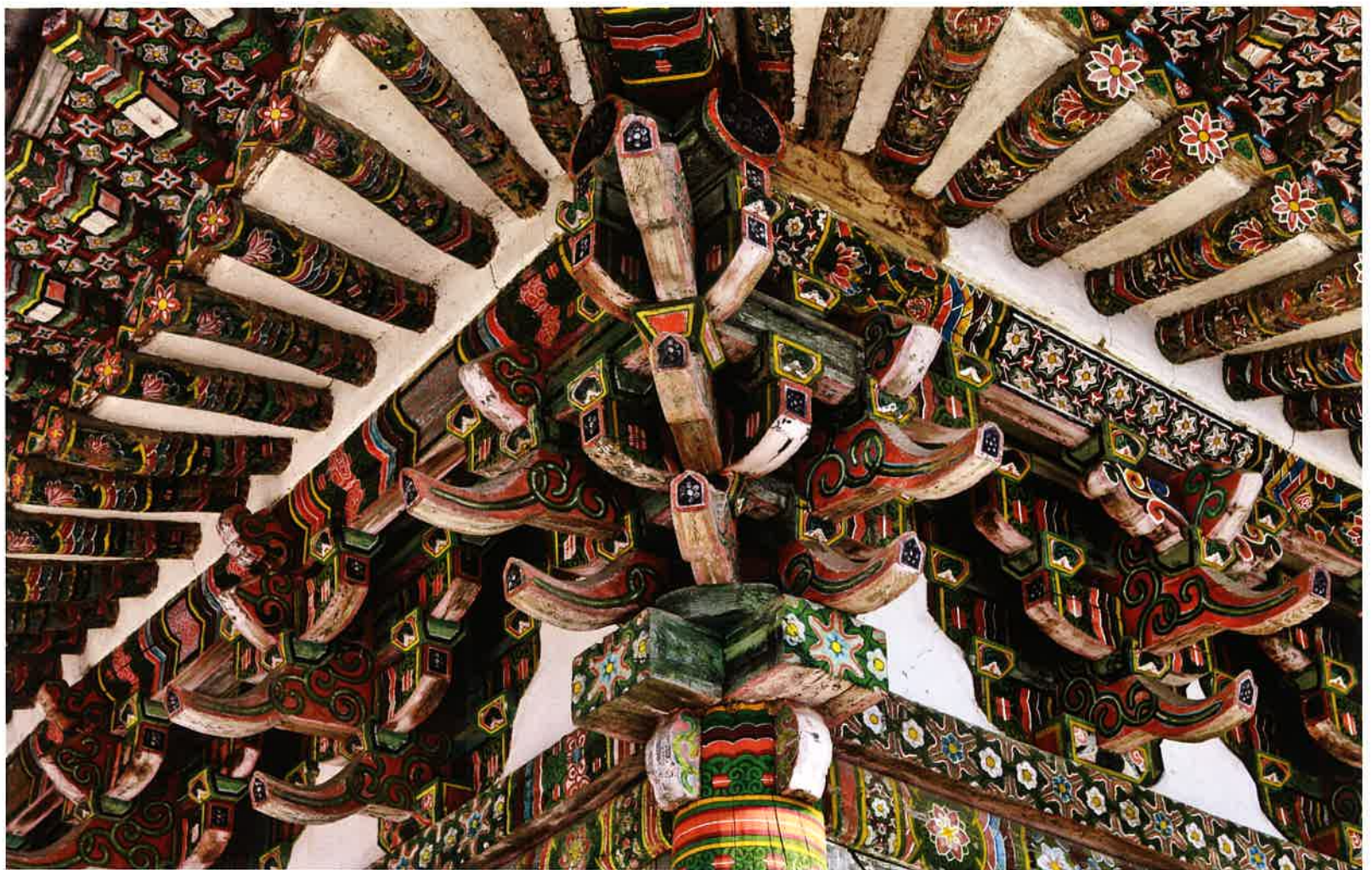
장경각 앞면 서쪽 귀포 / 藏經閣 前面 西側 耳包 / front western corner brackets, Changgyonggak hall
