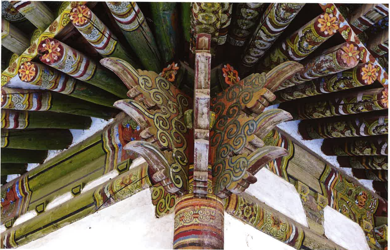
극락전 서쪽 뒷면 귀포 / 極樂殿 西側 後面 耳包 / western back corner brackets, Kūngnakchōn hall
