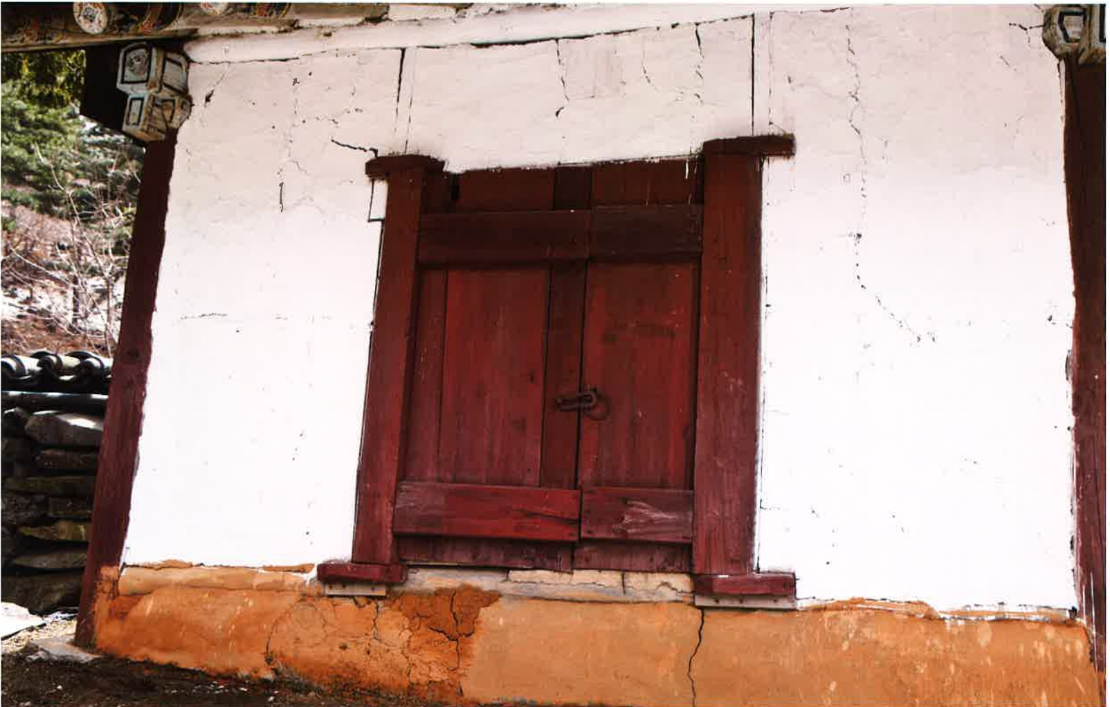
요사채 북쪽 벽체 / 寮舍齋 北側 壁體 / northern wall, priest's residence
