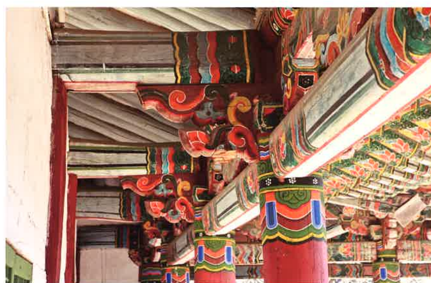
천주루 뒷간 내부 공포 / 天柱樓 退間 內部 栱包 brackets of space with extra poles outside the inner fence, Ch'ŏnjuru hall
