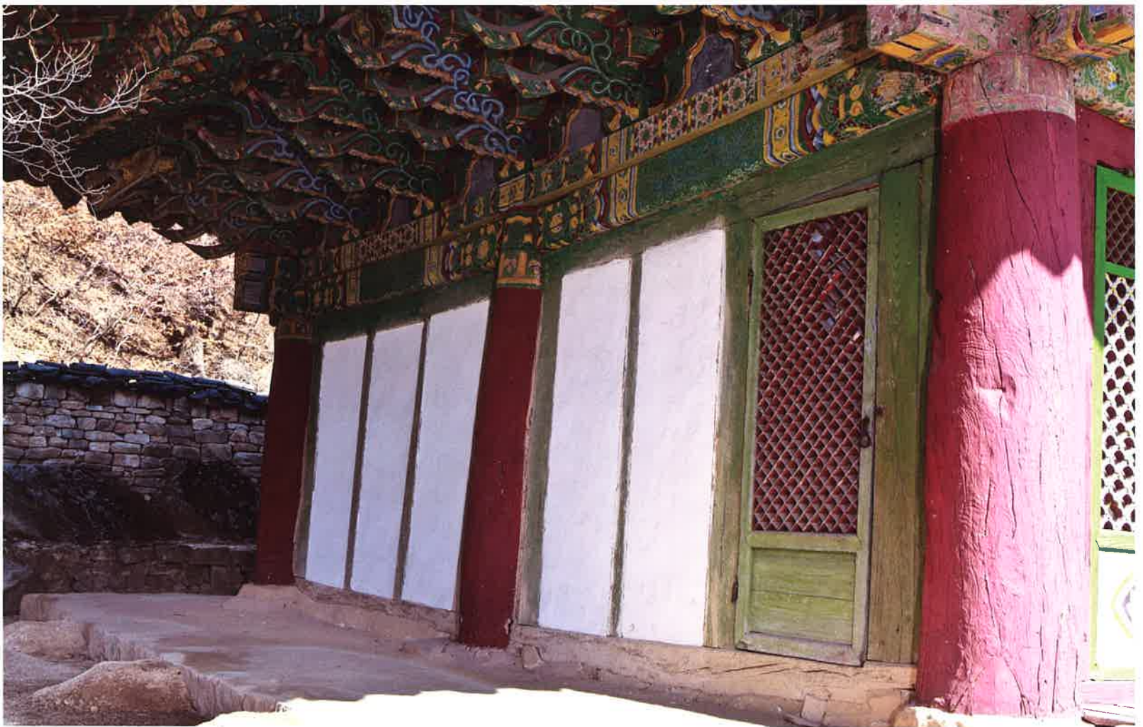
보광전 서쪽 벽체 / 普光殿 西側 壁體 / western wall, Pogwangjŏn hall
