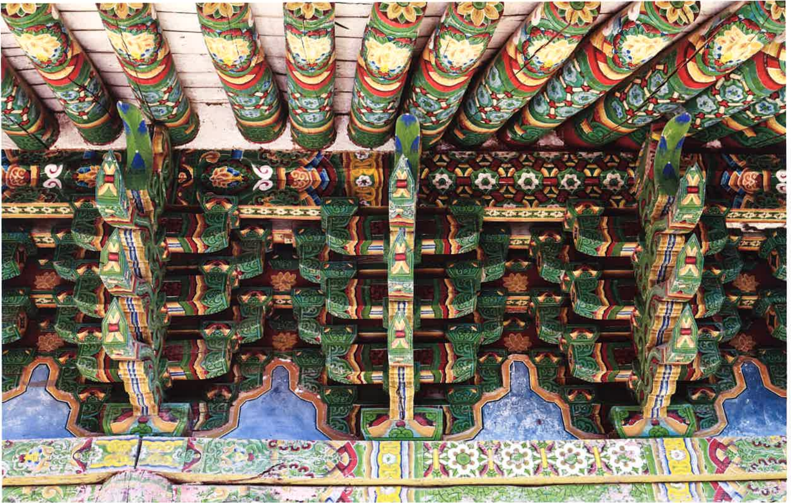
보광전 앞면 주간포 1 / 普光殿 前面 柱間包 1 / brackets 1 between front columns, Pogwangjon hall
