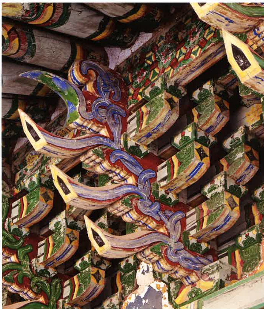
보광전 뒷면 주간포 / 普光殿 後面 柱間包 brackets between backward columns, Pogwangjŏn hall
