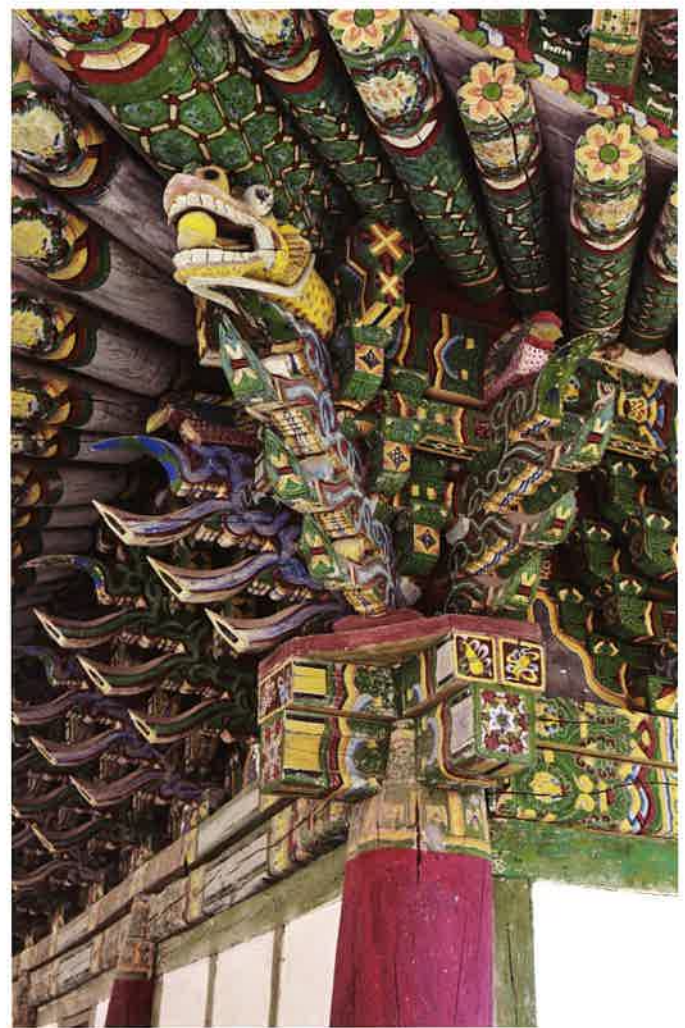
보광전 뒷면 서쪽 귀포 / 普光殿 後面 西側 耳包 backward western corner brackets, Pogwangjŏn hall
