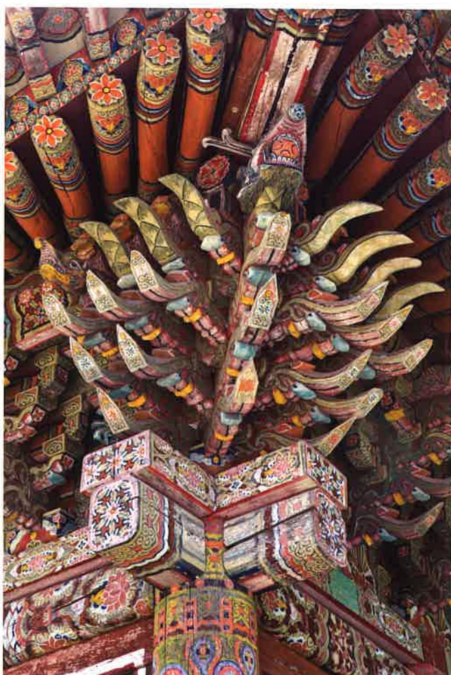
대웅전 앞면 동쪽 귀포 / 大雄殿 前面 東側 耳包 front eastern corner brackets, Taeungjŏn hall
