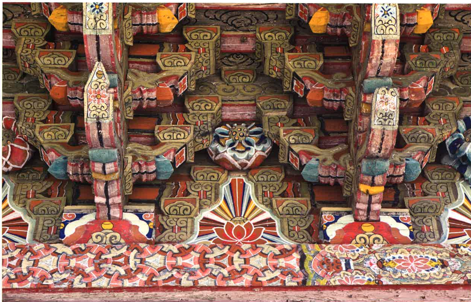
대웅전 앞면 주간포 / 大雄殿 前面 柱間包 / brackets between front columns, Taeungjŏn hall
