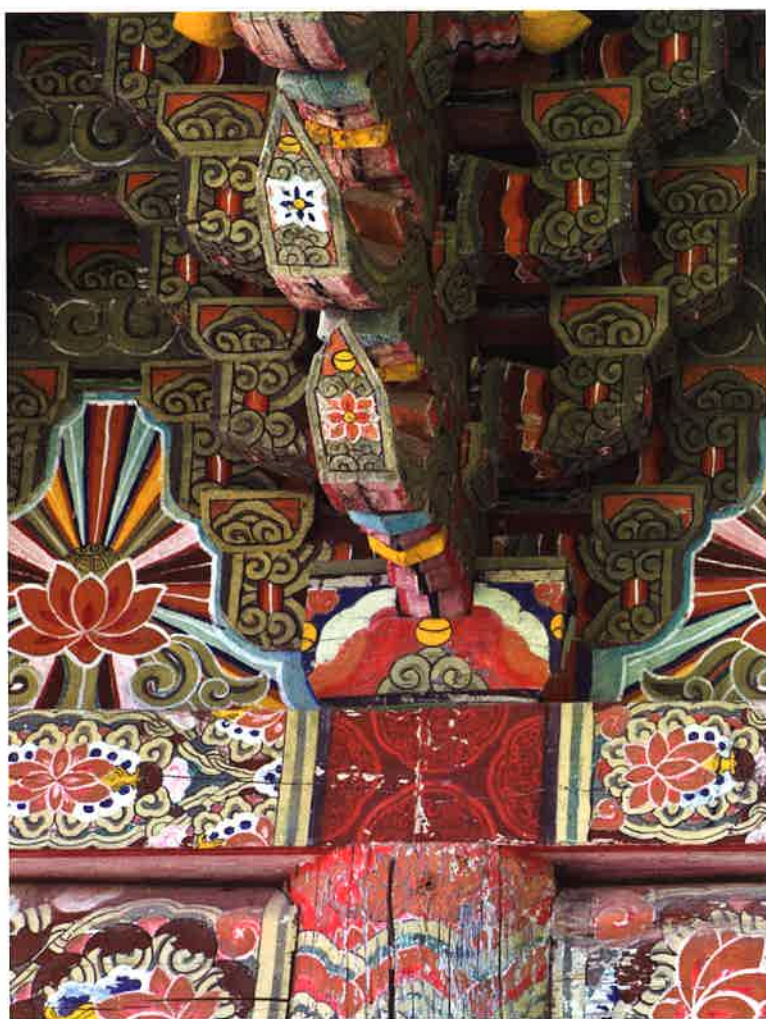
대웅전 동쪽 측면 주간포 / 大雄殿 東側 柱間包 brackets between eastern columns, Taeungjön hall
