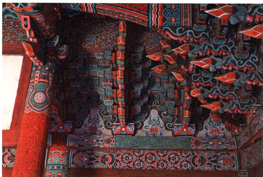
대웅전 뒷면 동쪽 귀포 / 大雄殿 後面 東側 耳包 backward eastern corner brackets, Taeungjeon hall
