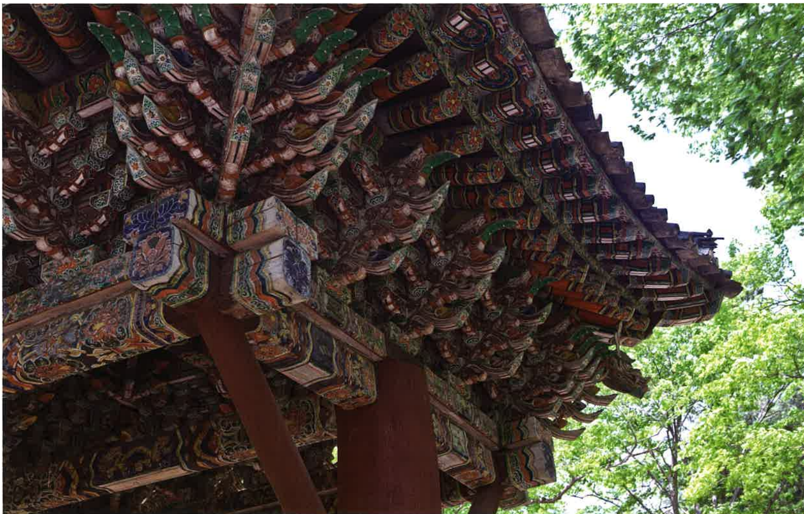
조계문 동쪽 귀포 / 曹溪門 東側 耳包 / eastern corner brackets, Chogyemun gate
