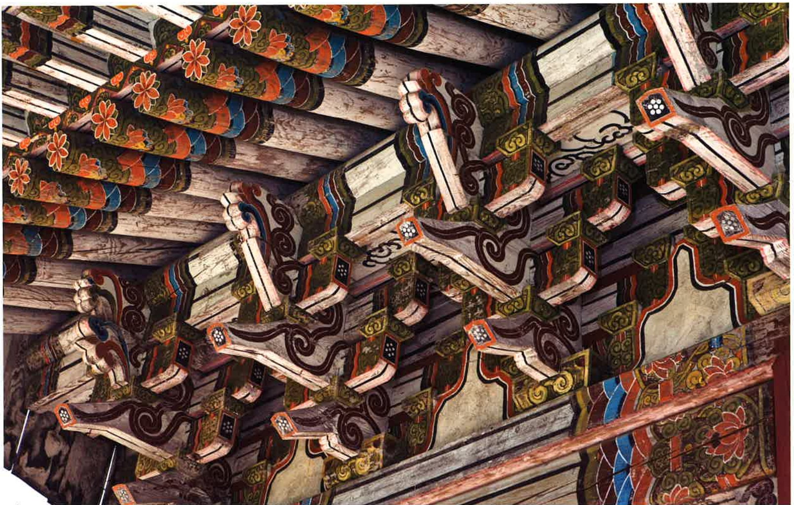
호지문 앞면 주간포 / 護持門 前面 柱間包 / front brackets between columns, Hojimun gate
