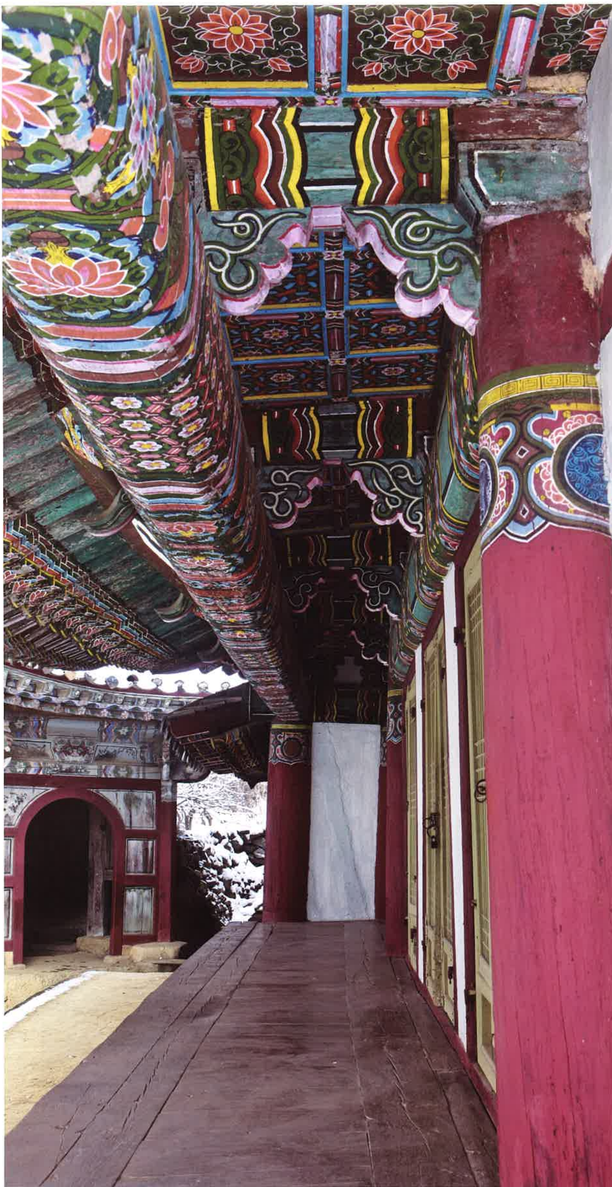
상원암 본전 뒷간 / 上院庵 本殿 退間 a space with extra poles outside the inner fence of main hall, Sangwŏnam
