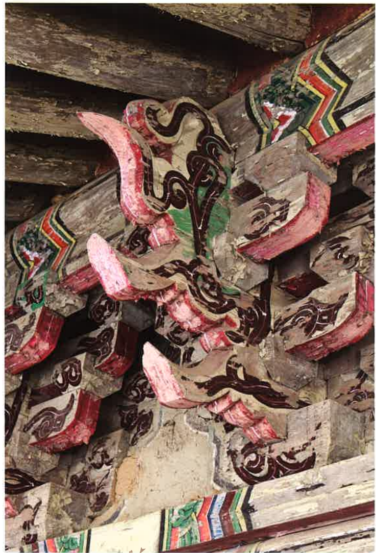
칠성각 뒷면 귀포 / 七星閣 後面 耳包 corner brackets of backward side, Ch'ilsönggak shrine
