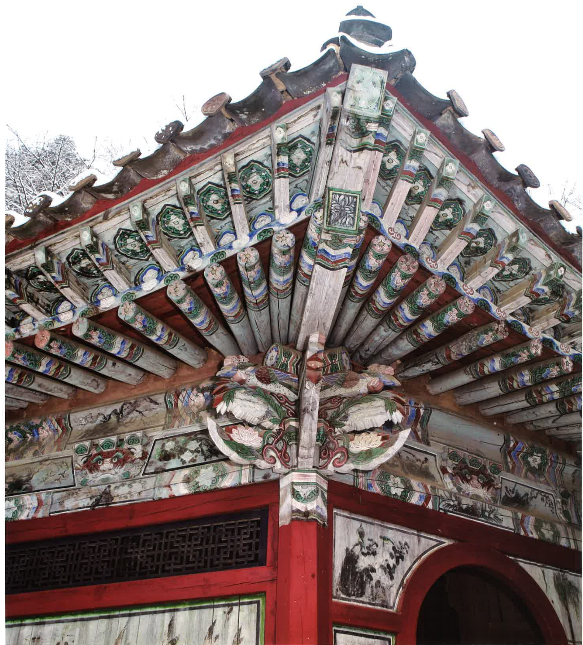
상원암 수각 추녀 / 上院庵 水閣 春舌 / protruding corners of eaves, pavilion on the water, Sangwónam
