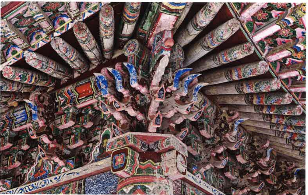
칠성각 앞면 동쪽 귀포 / 七星閣 前面 東側 耳包 front eastern corner brackets, Ch'ilsönggak shrine
