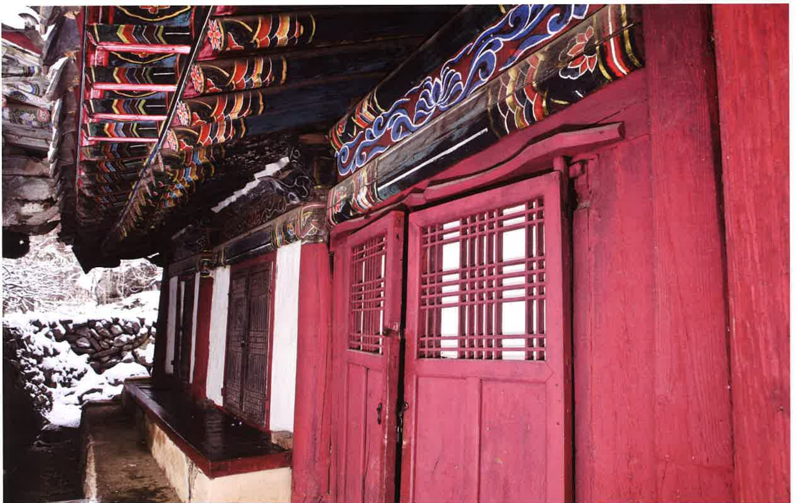
상원암 본전 서쪽 날개채 앞면 / 上院庵 本殿 西側 翼舍 前面 / front of western wing building of main hall, Sangwŏnam
