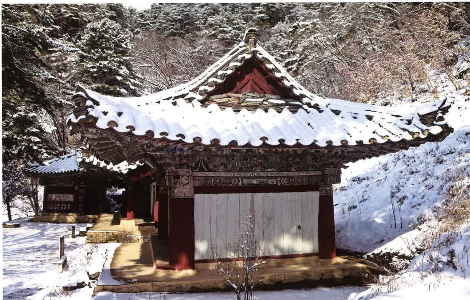
칠성각 동쪽 측면 / 七星閣 東側面 / eastern side, Ch'ŏlsŏnggak shrine
