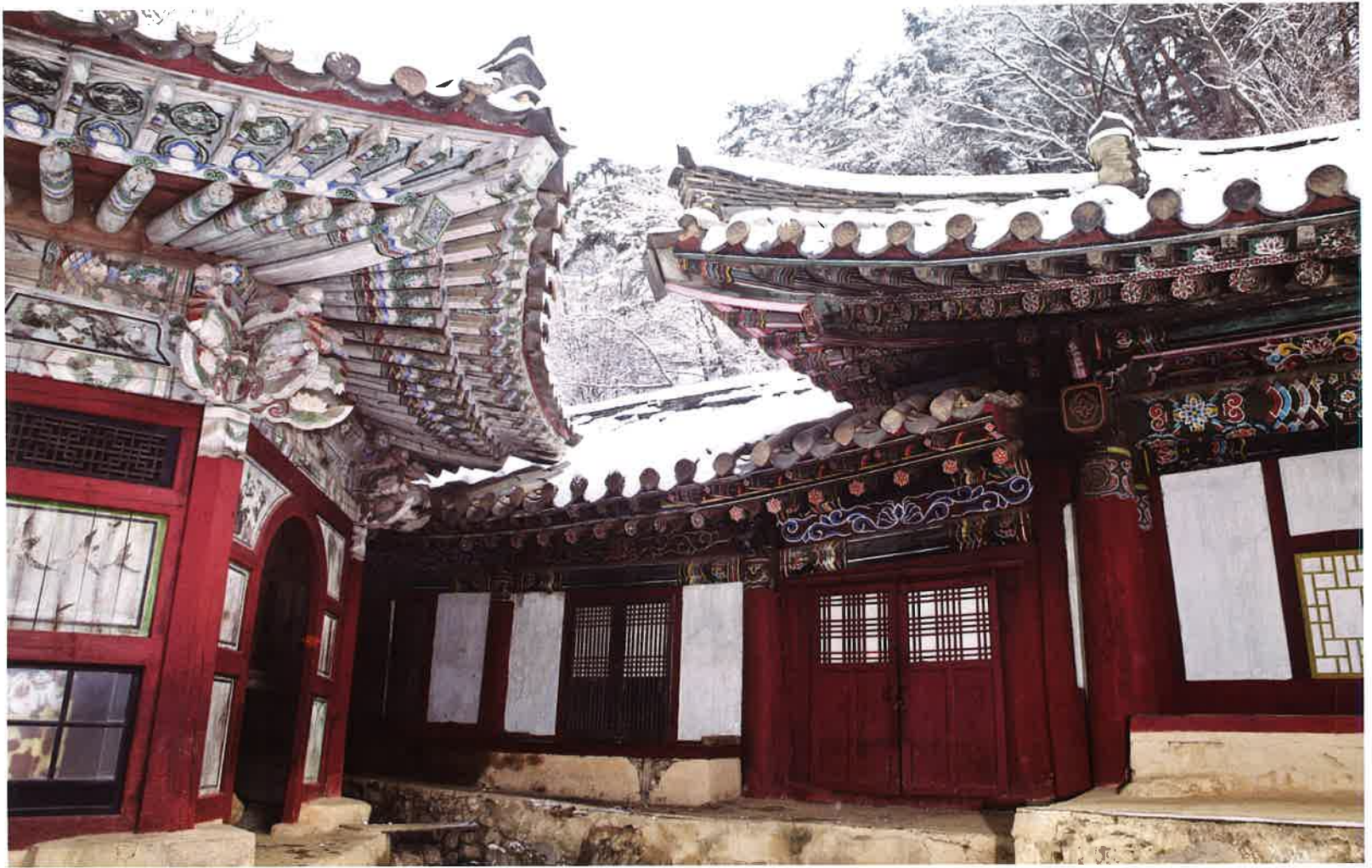
상원암 본전 서쪽 날개채 / 上院庵 本殿 西側 翼舍 / western wing building of main hall, Sangwŏnam
