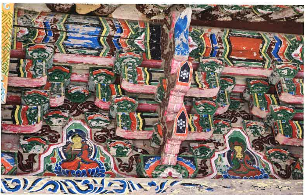
칠성각 앞면 주간포 / 七星閣 前面 柱間包 brackets between front columns, Ch'ilsönggak shrine
