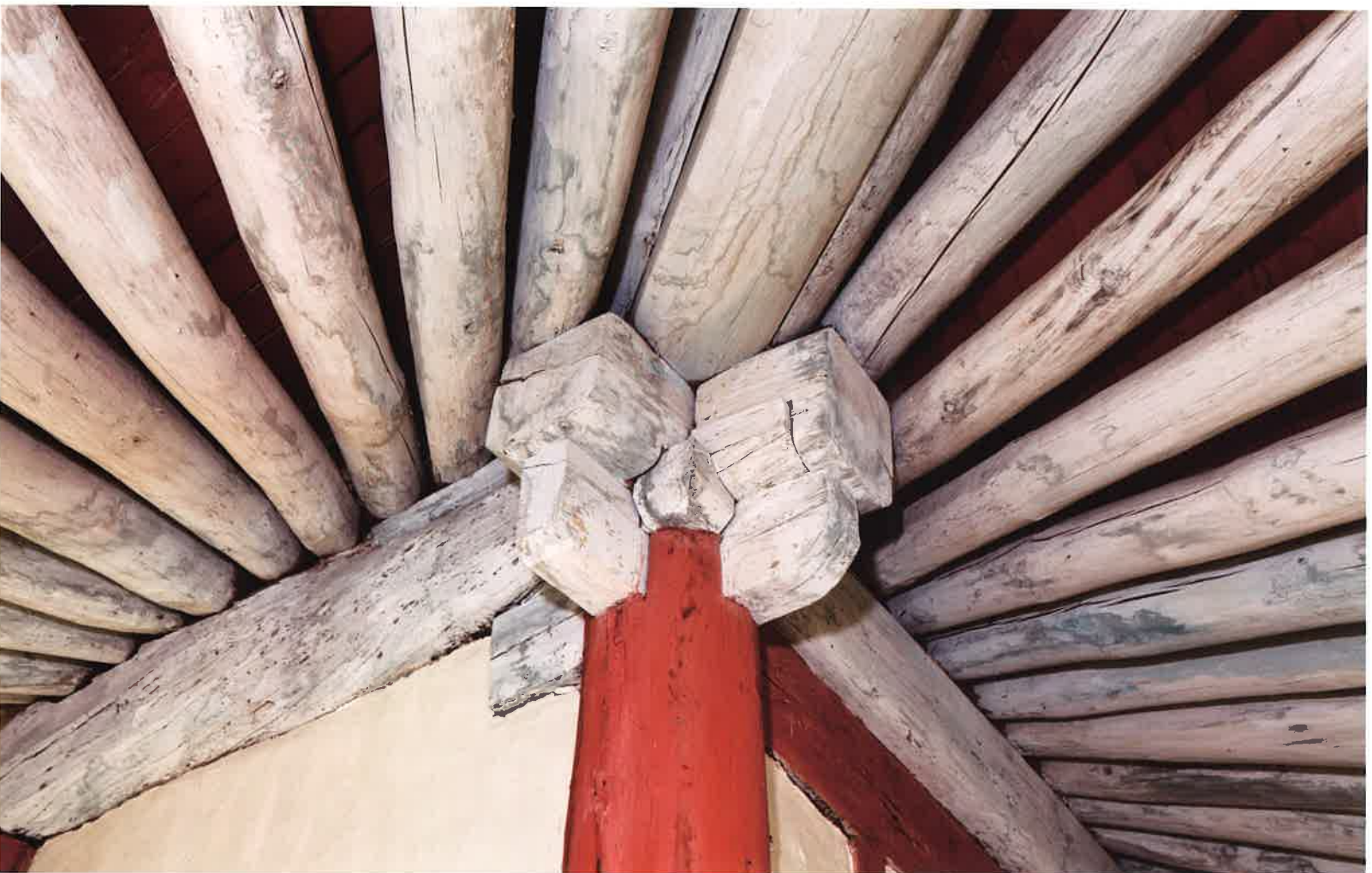
화장암 뒷면 귀포 / 華藏庵 後面 耳包 / backward corner brackets, Hwajangam
