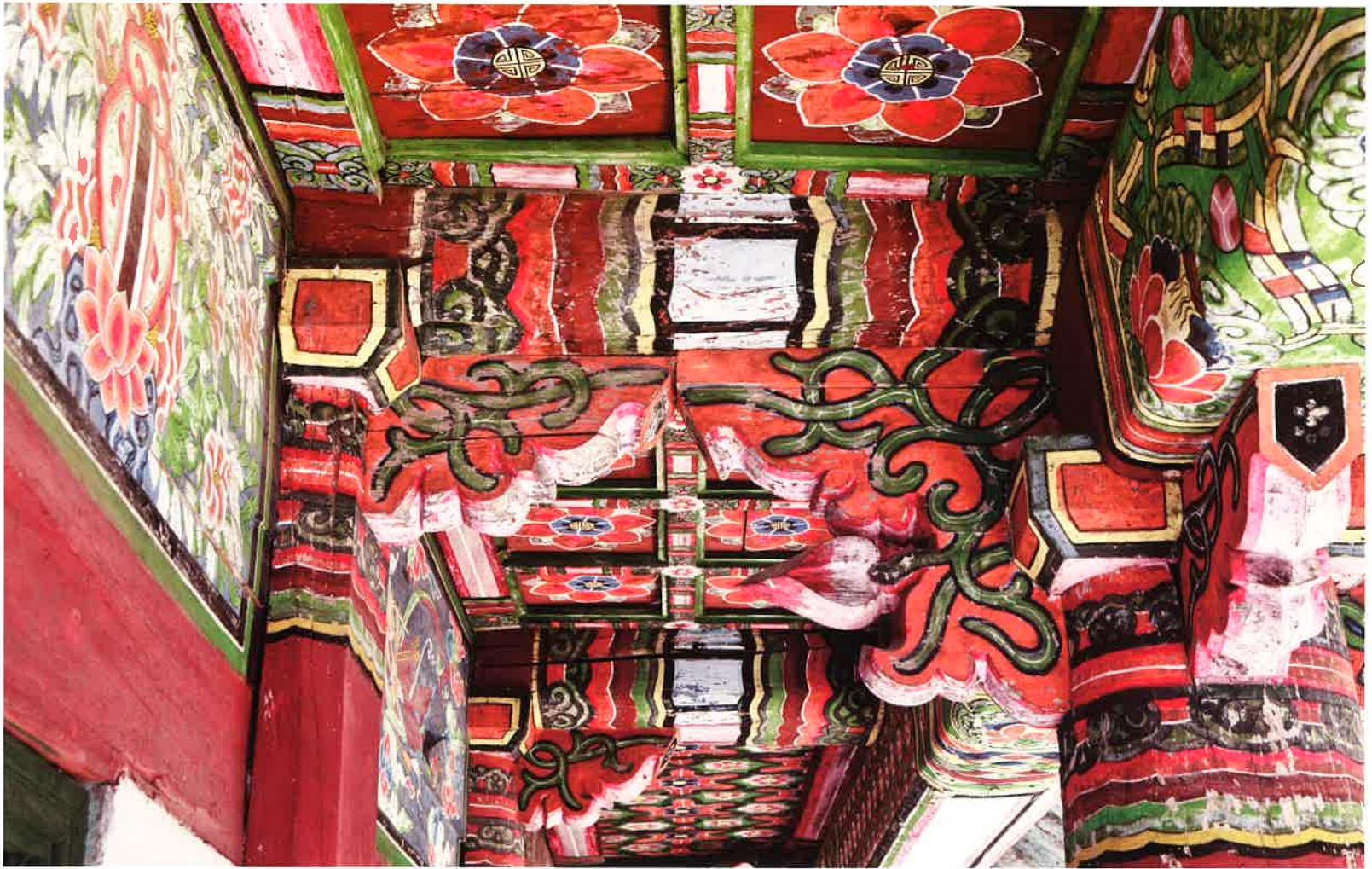
화장암 틈간 공포 / 華藏庵 退間 拱包 brackets of space with extra poles outside the inner fence, Hwajangam
