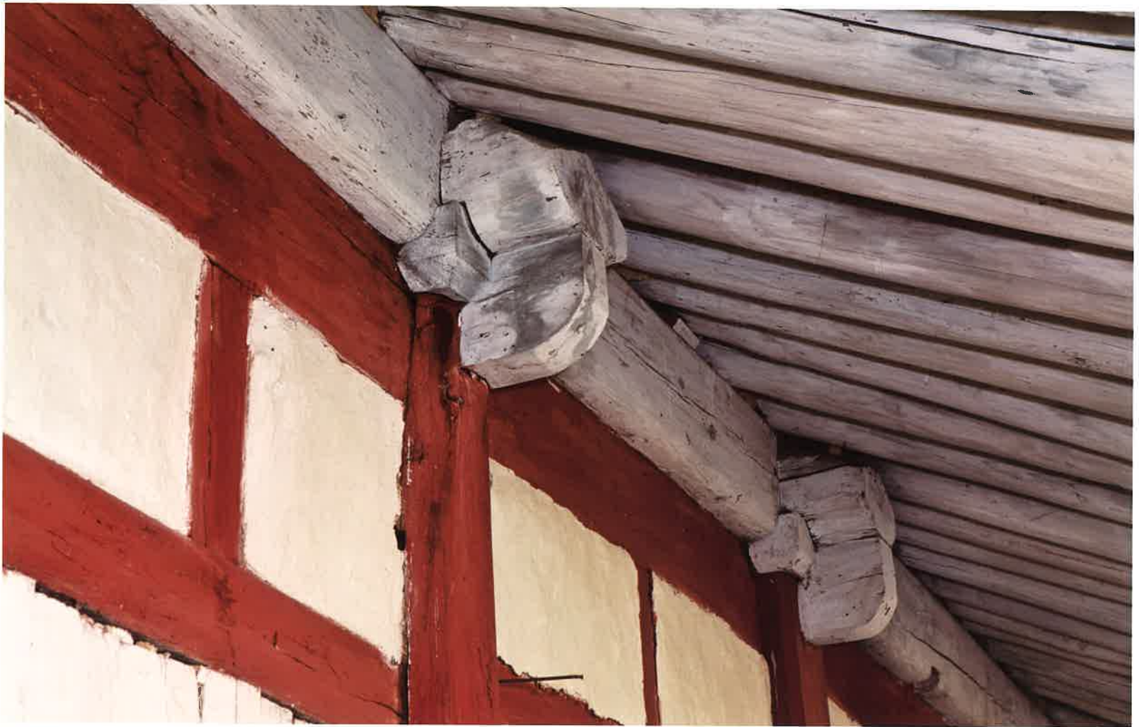
화장암 뒷면 주상포 / 華藏庵 後面 柱上包 / brackets above backward columns, Hwajangam
