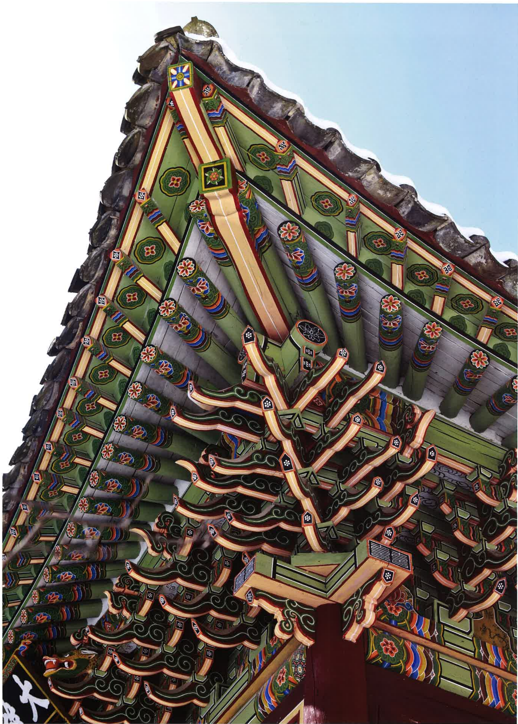
대웅전 앞면 동쪽 추녀와 사례 / 大雄殿 前面 東側 春舌・蛇羅 / eastern protruding corners of eaves and rafters, Taungjeon hall
