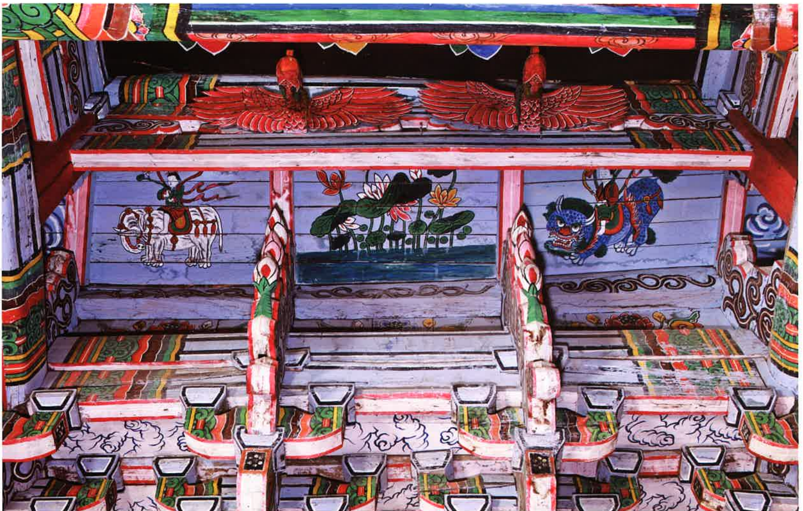
대웅전 내부 빗반자 별화 / 大雄殿 内部 斜天障 別畫 / attached painting on inclined ceiling, Taeungjŏn hall
