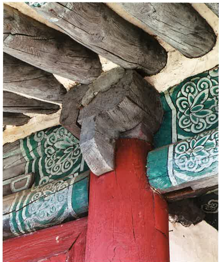
요사채 앞면 귀포 / 寮舍寨 前面 耳包 front corner brackets, priest's residence
