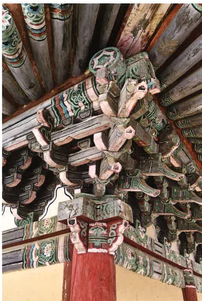
극락보전 뒷면 서쪽 귀포 / 極樂寶殿 後面 耳包 backward western corner brackets, Kŭngnakpojŏn hall
