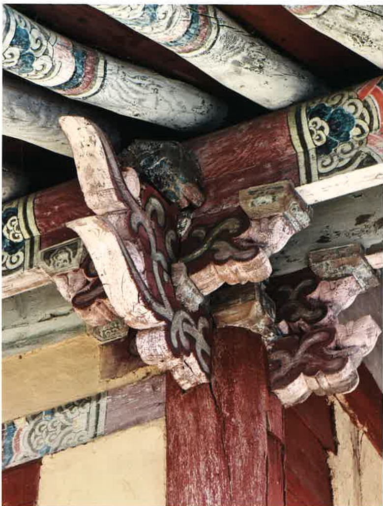
명부전 앞면 귀포 / 冥府殿 前面 耳包 front corner brackets, Myōngbujōn hall
