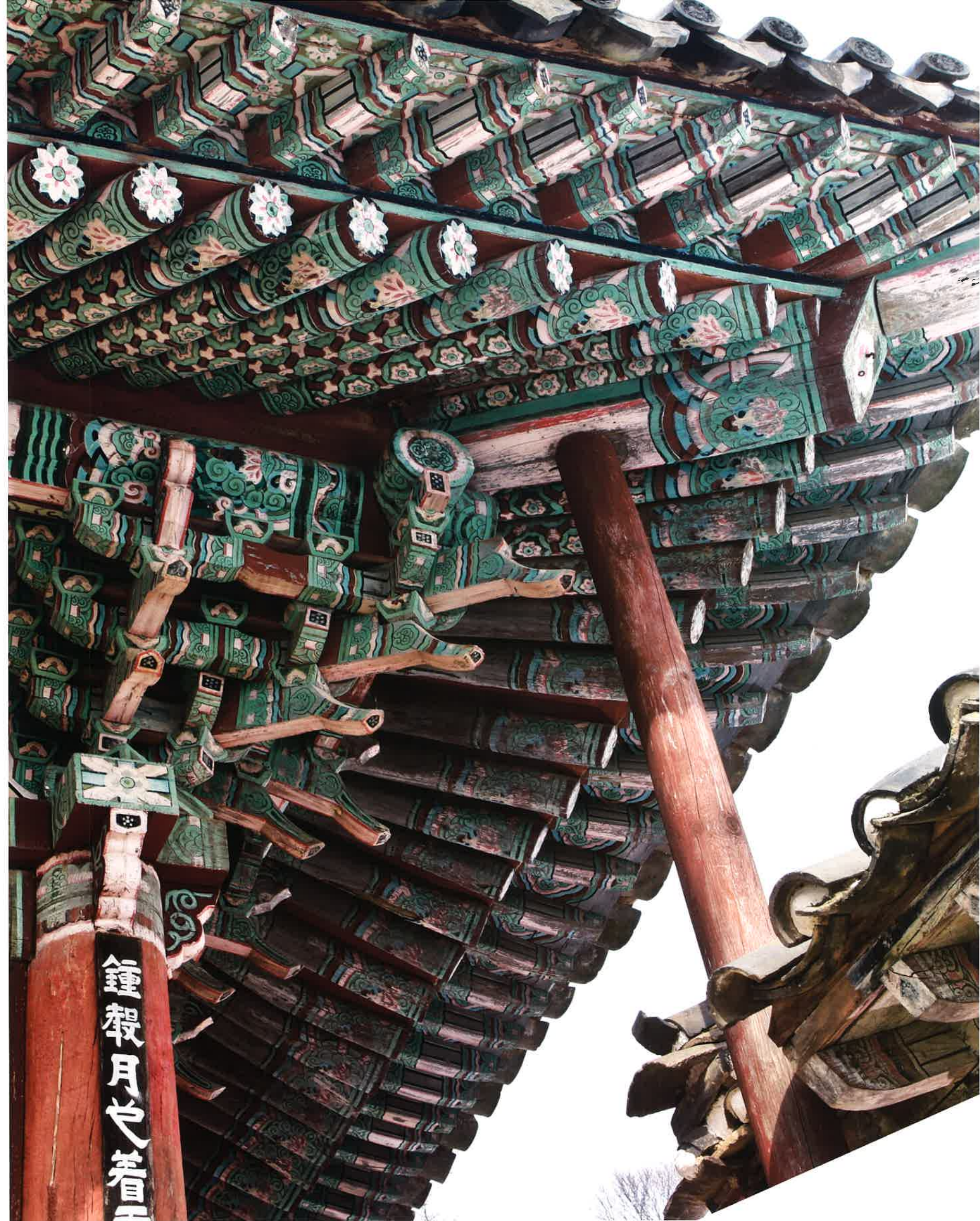
극락보전 앞면 동쪽 귀포와 활주 / 極樂寶殿 前面 東側 耳包·活柱 / eastern corner brackets and brace, Kŭngnakpojŏn hall
