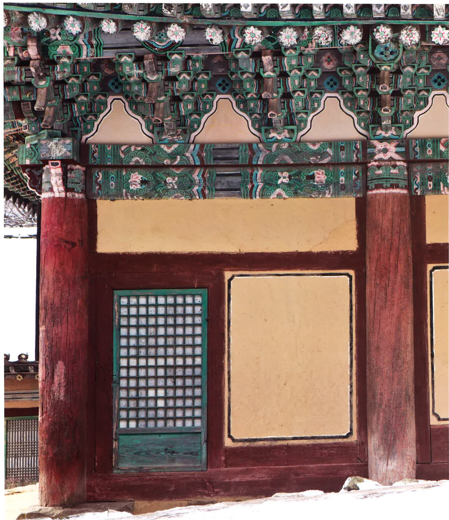
극락보전 동쪽 측면 창호 / 極樂寶殿 東側 窓戶 / eastern wall and door, Kŭngnakpojŏn hall
