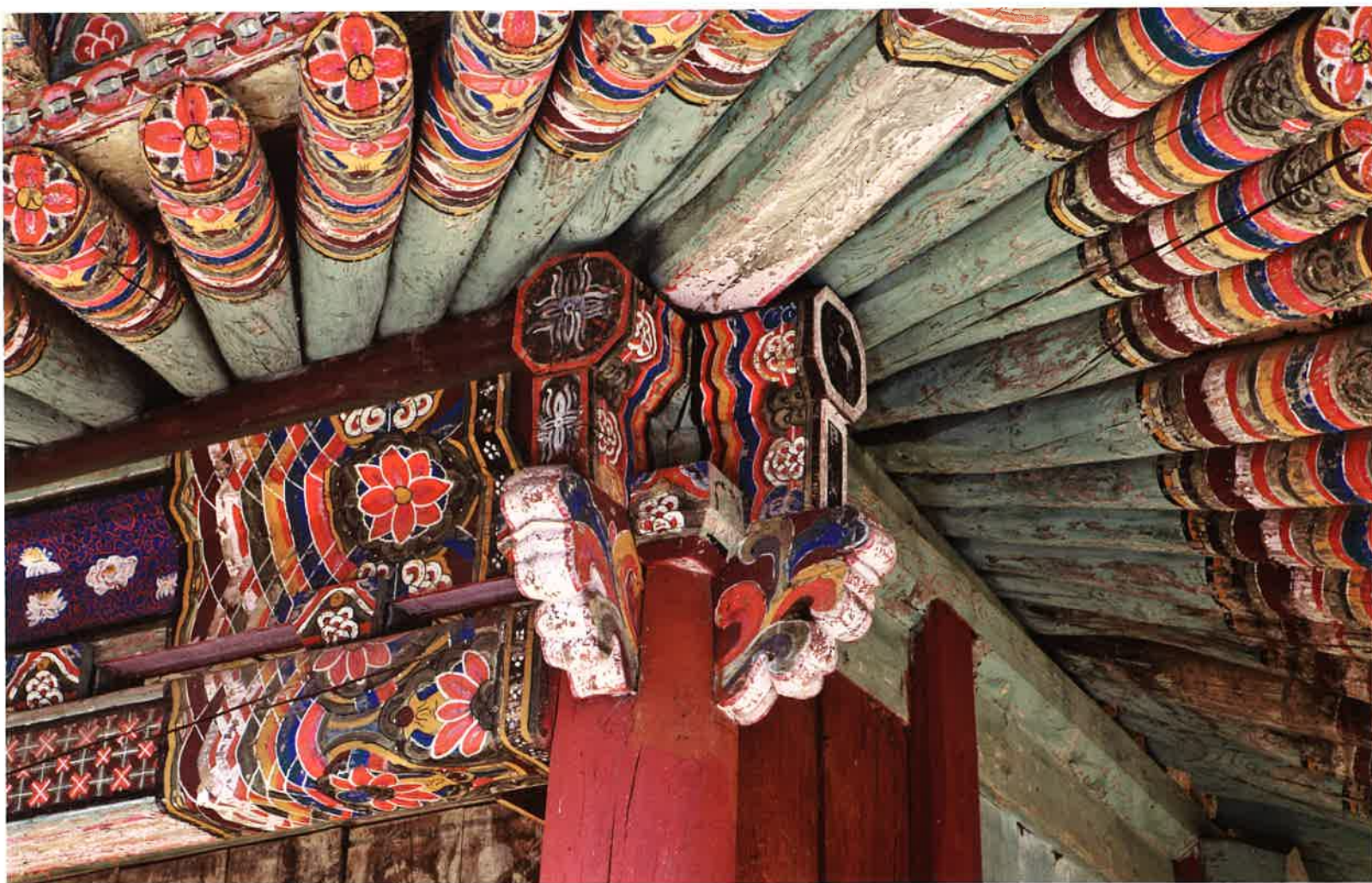
극락전 동쪽 측면 귀포 / 極樂殿 東側 耳包 / eastern brackets, Paekhwajŏn hall
