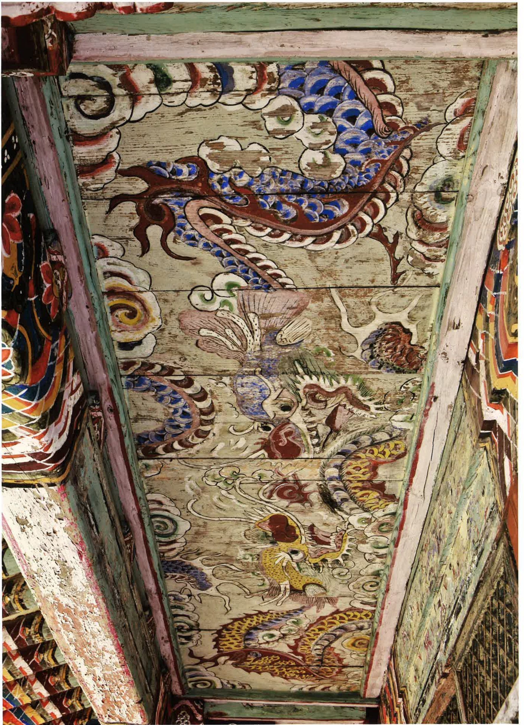
극락전 뒷간 반자 별화 1 / 極樂殿 退間 天障 別畫 1 / attached painting 1 on ceiling of space with extra poles outside the inner fence, Kūngnakjŏn hall
