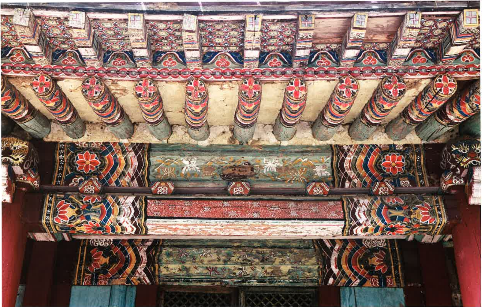
극락전 앞면 액방과 도리·장혀 1 / 極樂殿 前面 額枋, 道里·長舌 1 front lintel, strip of wood supporting a beam 1, Kūngnakjŏn hall
