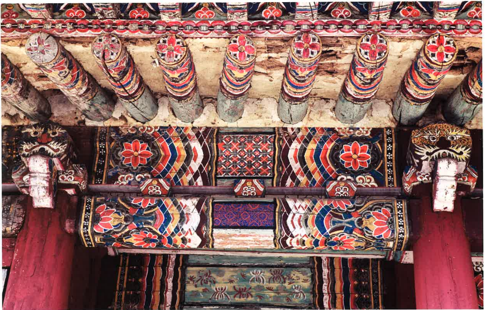
극락전 앞면 액방과 도리·장혀 3 / 極樂殿 前面 額枋·道里·長舌 3 / front lintel, strip of wood supporting a beam 3, Kŭngnakjŏn hall
