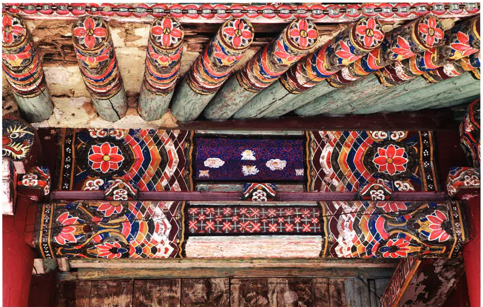
극락전 앞면 액방과 도리·장혀 2 / 極樂殿 前面 額枋, 道里·長舌 2 front lintel, strip of wood supporting a beam 2, Kūngnakjŏn hall
