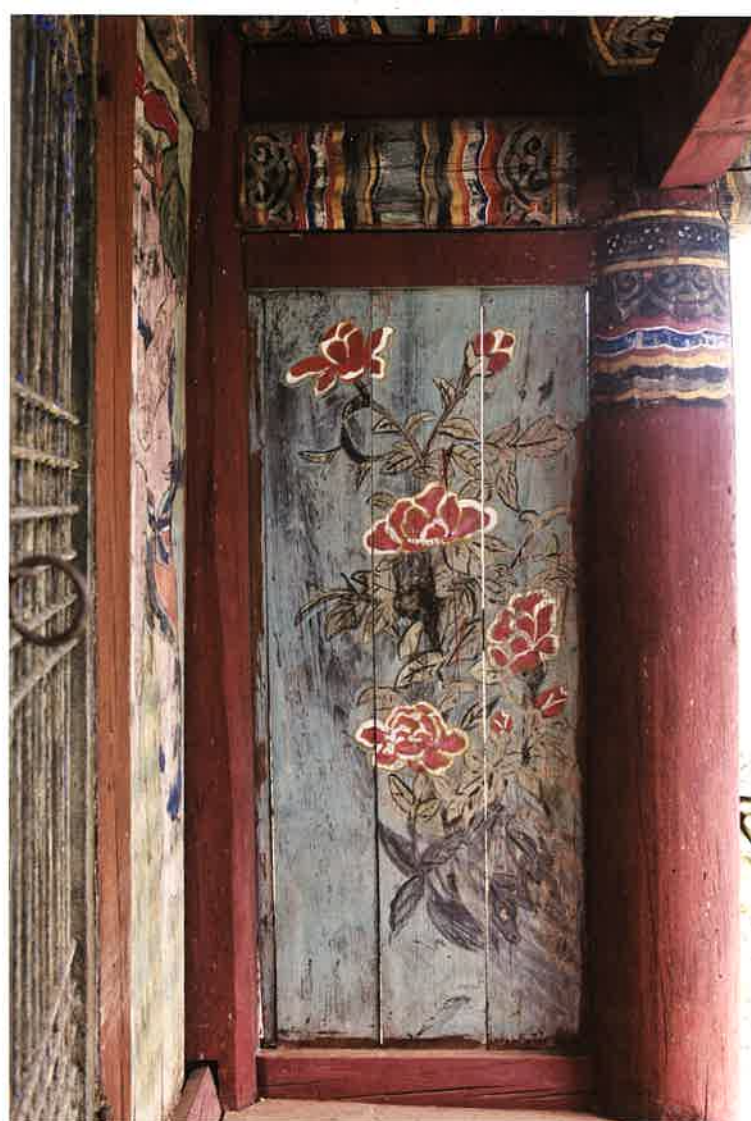
칠성각 뒷간 오른쪽 별화 / 七星閣 退間 右側 別畵 attached painting on the right side of a space with extra poles outside the inner fence, Ch'ilssonggak shrine
