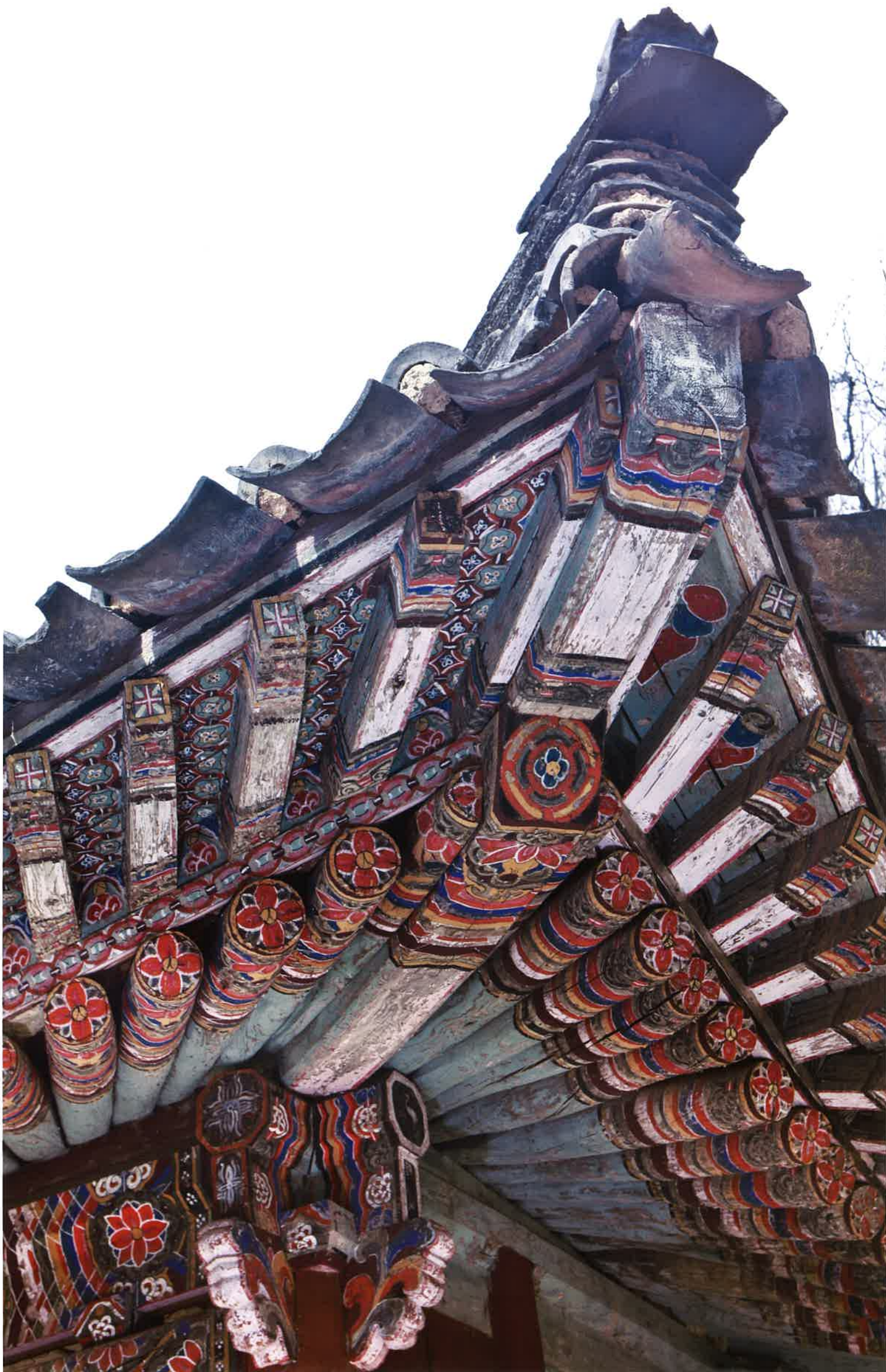
극락전 앞면 추녀와 사래 / 極樂殿 前面 春舌·蛇羅 front protruding corners of eaves and rafters, Kūngnakjŏn hall
