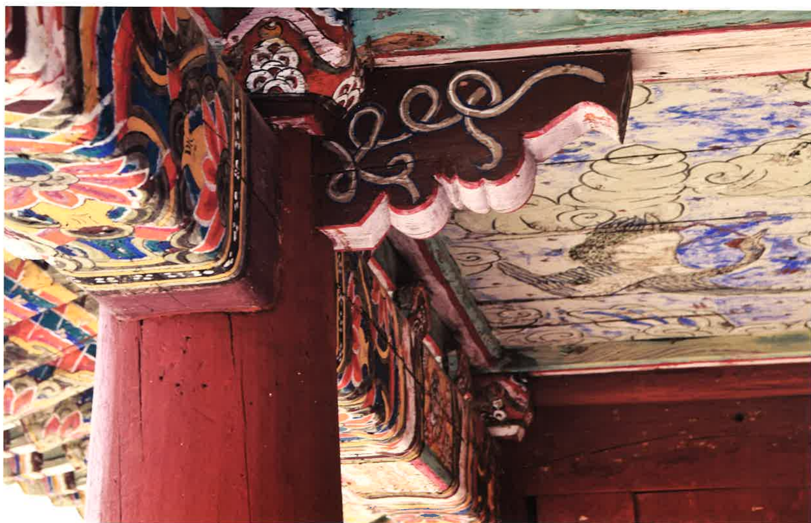
극락전 뒷간 기둥과 액방 / 極樂殿 退間 平柱·額枋 / columns and lintel of space with extra poles outside the inner fence, Kŭngnakjŏn hall
