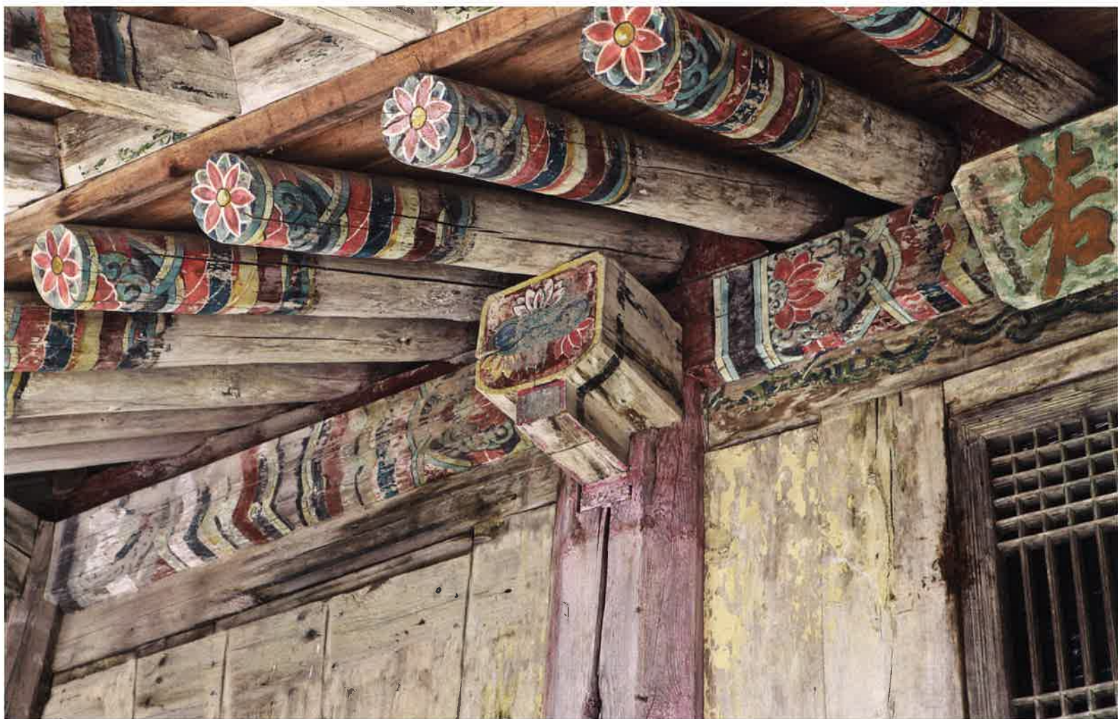
법왕대 앞면 주간포 / 法王臺 前面 柱間包 / brackets between front columns, Pöbwangdae
