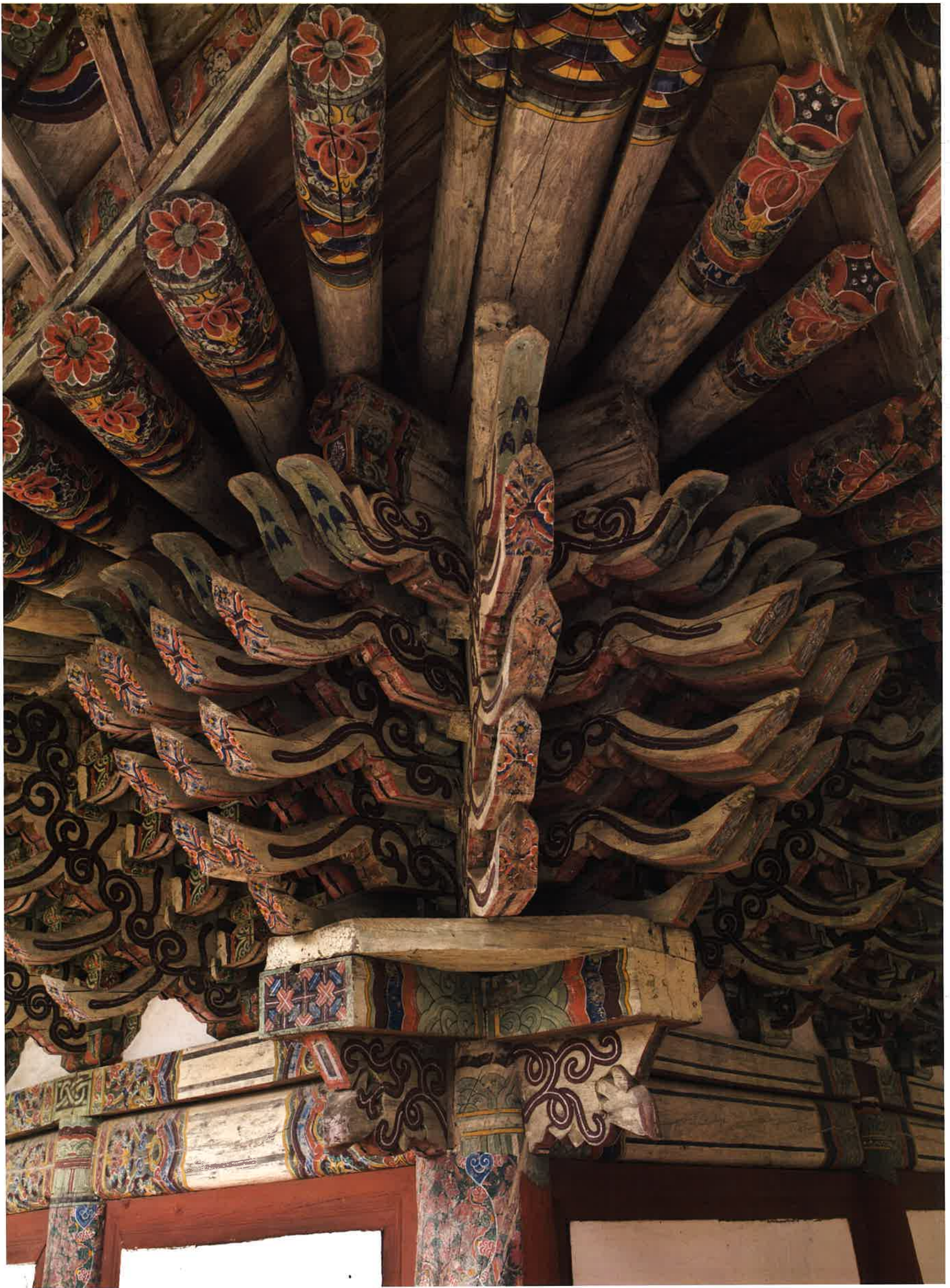
대웅전 뒷면 동쪽 귀포 / 大雄殿 後面 東側 耳包 / backward eastern corner brackets, Taungjeon hall
