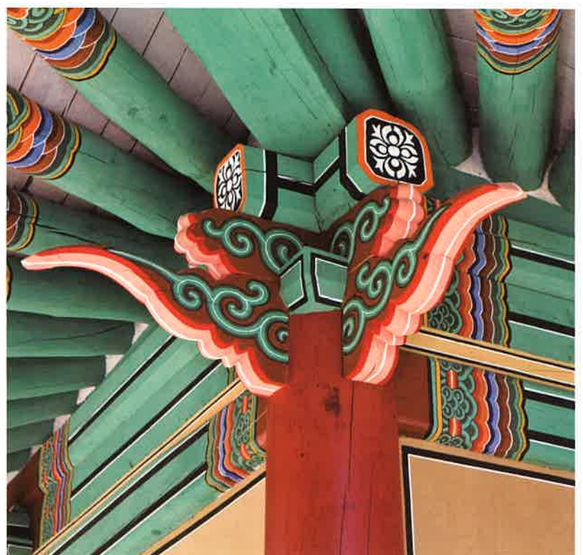
무량수각 뒷면 서쪽 귀포 / 無量壽閣 後面 西側 耳包 backward western corner brackets, Muryangsugak hall
