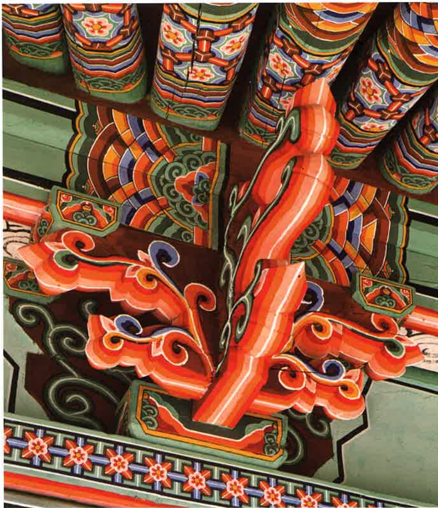
대웅전 동쪽 측면 주간포 / 大雄殿 東側 柱間包 brackets between eastern columns, Taeungjeon hall
