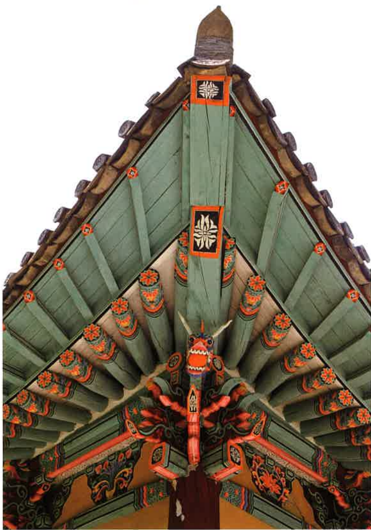
극락전 앞면 서쪽 추녀 / 極樂殿 前面 西側 春舌 western protruding corners of eaves, Kūngnakjŏn hall
