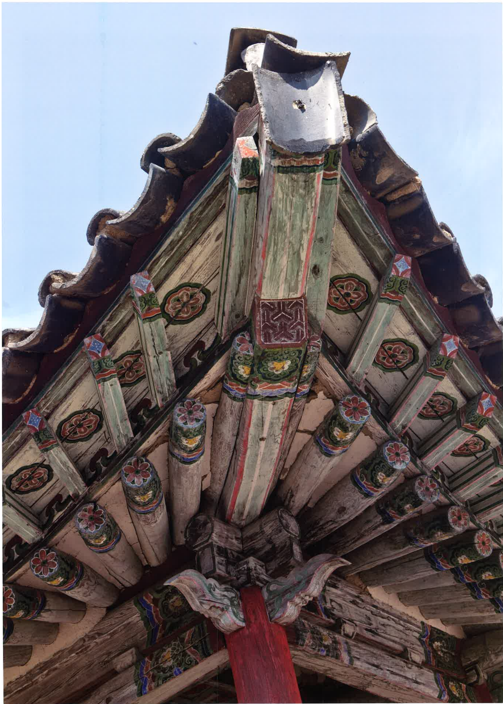
애월루 동쪽 추녀와 사래 / 愛月樓 東側 春舌·蛇羅 / eastern protruding corners of eaves and rafters, Aewöllu
