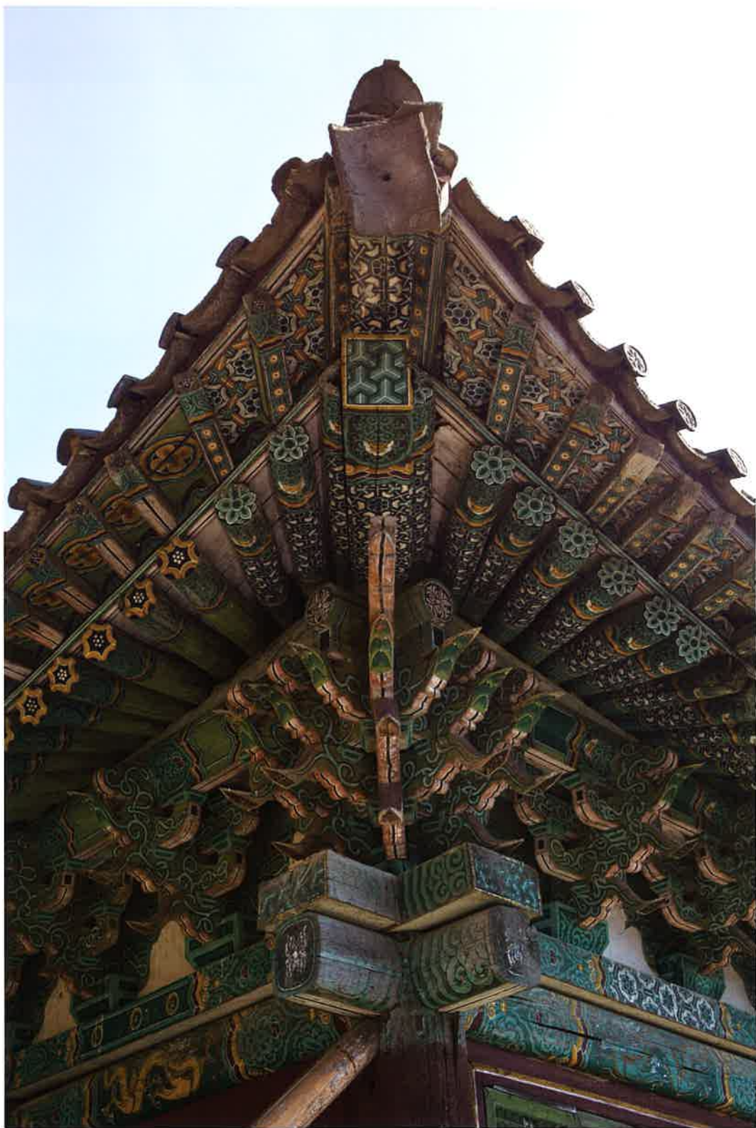
대웅전 앞면 서쪽 추녀와 사래 / 大雄殿 前面 西側 春舌·蛇羅 front western protruding corners of eaves and rafters, Taeungjŏn hall
